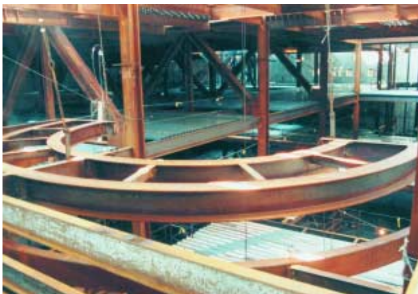
Circular stair on north side of building.
