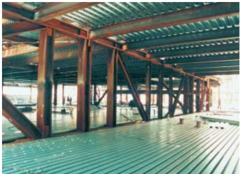
Vierendeel openings in story-high truss.
