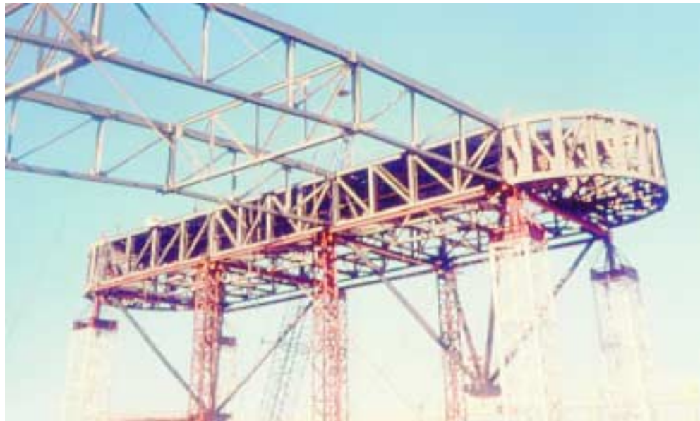
When the temporary erection columns are removed, the center "box" structure will support overhead scoreboards and other electrical equipment and rigging.
