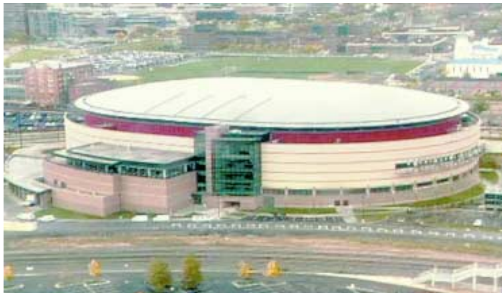
View of the completed Pepsi Center.
