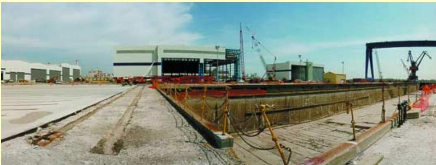
Site view: Panel and Fabrication shops to the far left, Grand Block shop in the center, and Paint Shop to the right. Goliath crane is also to the right, and the existing dry dock is in the foreground.
