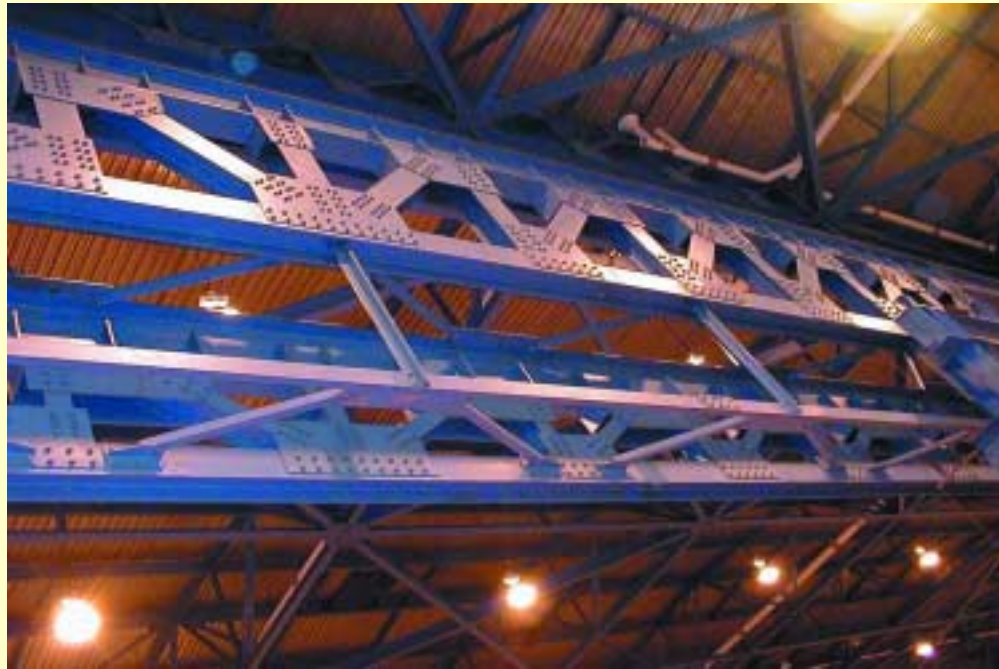
Larger spans utilized W14 chord and web members with field bolted connections to speed erection.
