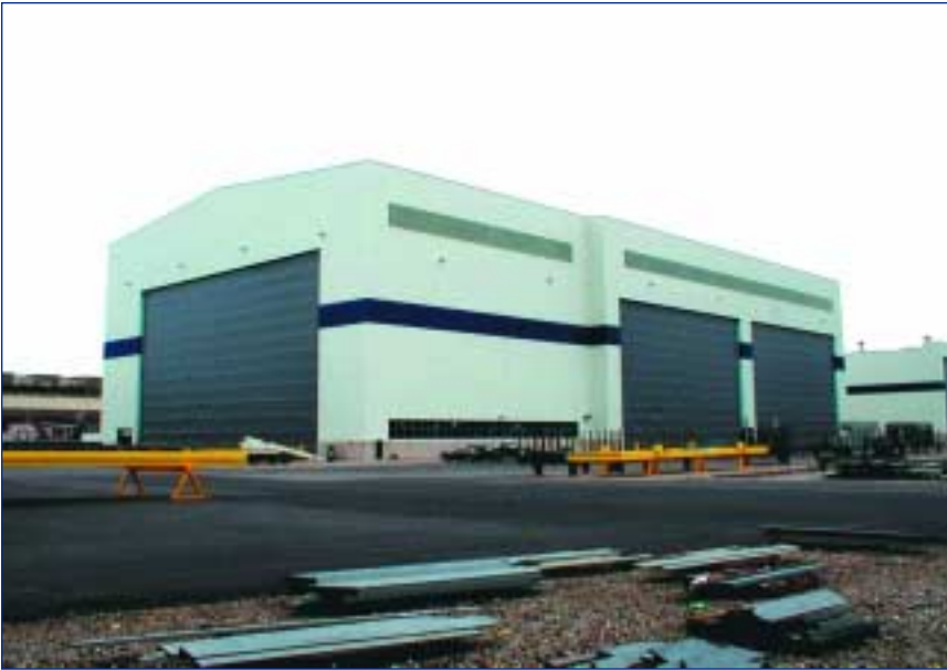
The exterior of the grand block is clad with cmu and prefinished metal panels.
