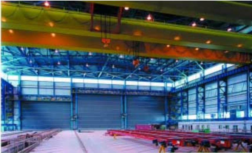
View inside Panel shop showing fabric doors, overhead trusses and bracing.
