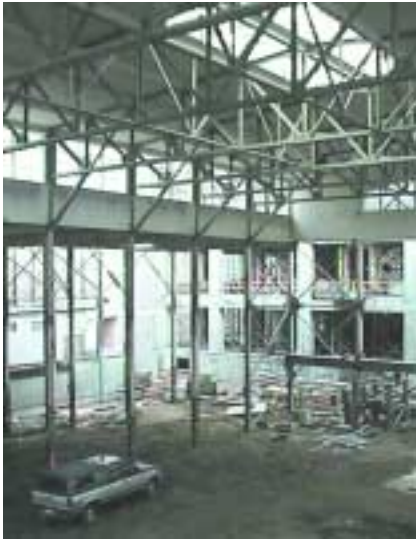
Interior of the Public market building showing the remaining structure after demolition of the existing second level and basement.
