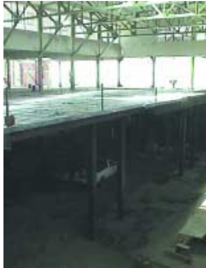
Interior view after installation of new second floor steel and steel deck.
