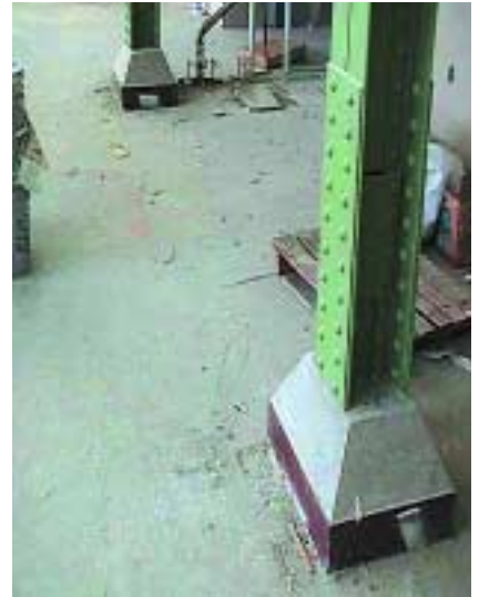
Columns cleaned and painted with intumescent paint. Bases have been grouted and the shoes and bolts hidden under a concrete cover.
