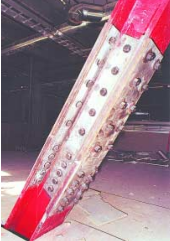
Slotted bolted prop connection.
