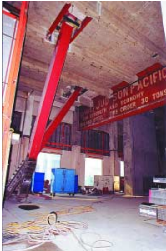
The new and the old: props appear alongside a 1930s vintage riveted steel transfer girder.
