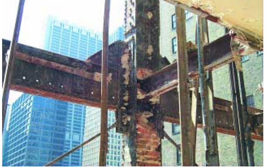
The exposed steel frame at the south building line of the Butler Building. Diagonal tension rods below the spandrel and extended end-plate connections of the spandrel, provide wind bracing for the 1924 structure.
