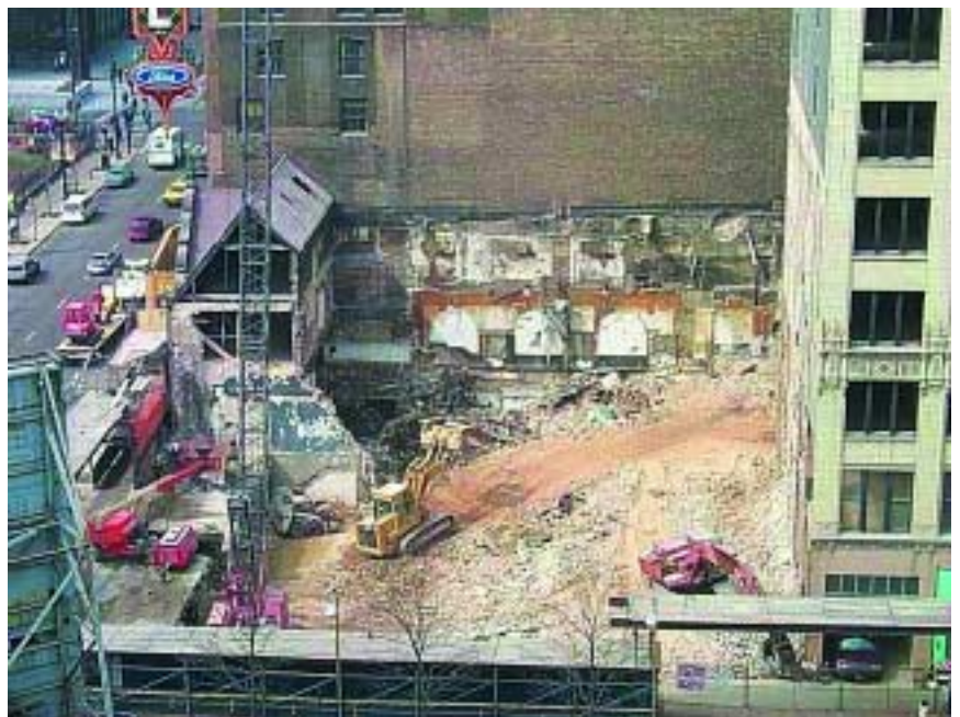
The site of the new 17-story building, after demolition of the existing low-rise building. The 1924 Butler Building on the right (north) and the southernmost bay of the Old Heidelberg (left) remain.
