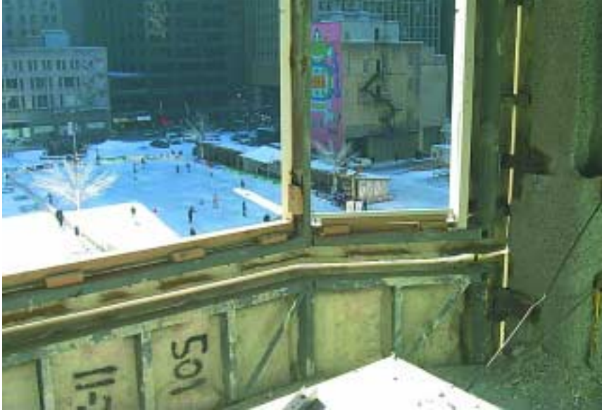
The GFRC panels were reinforced with lightweight steel studs and/or structural tube sections and were connected to the building columns.
