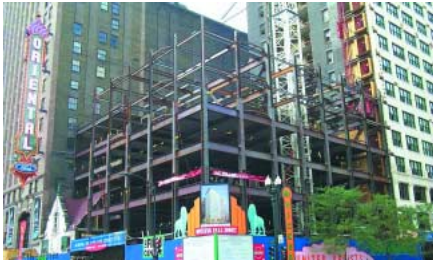
The new steel frame erected over and through the Old Heidelberg at the corner of the site.
