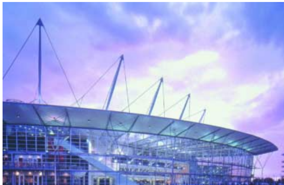
Exterior of Sydney SuperDome.
