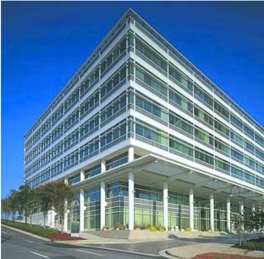
The Wachovia Building in North Carolina is an example of a successfully detailed curtain wall system.
