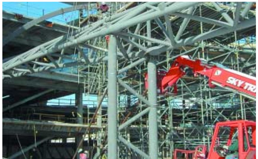
Naperville lobby roof truss and entry arch. Roof rafters in progress
