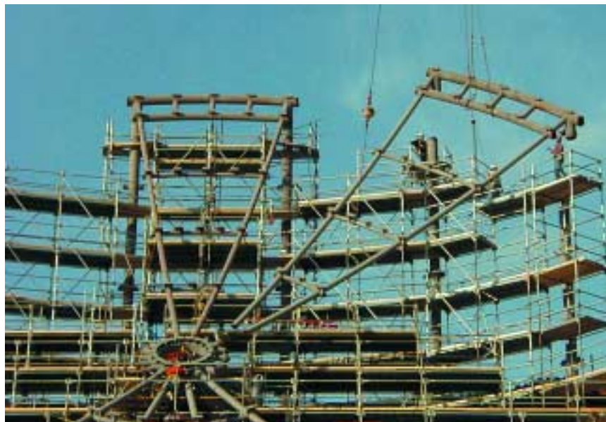
Lisle lobby roof "pie" segment being erected
