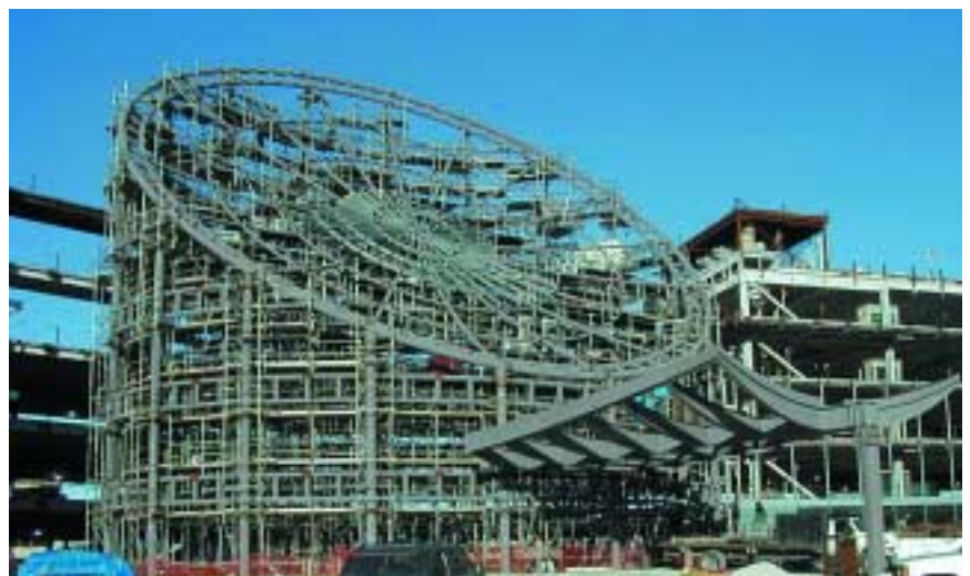
Lisle lobby and entry canopy framing with temporary erection scaffolding inside lobby
