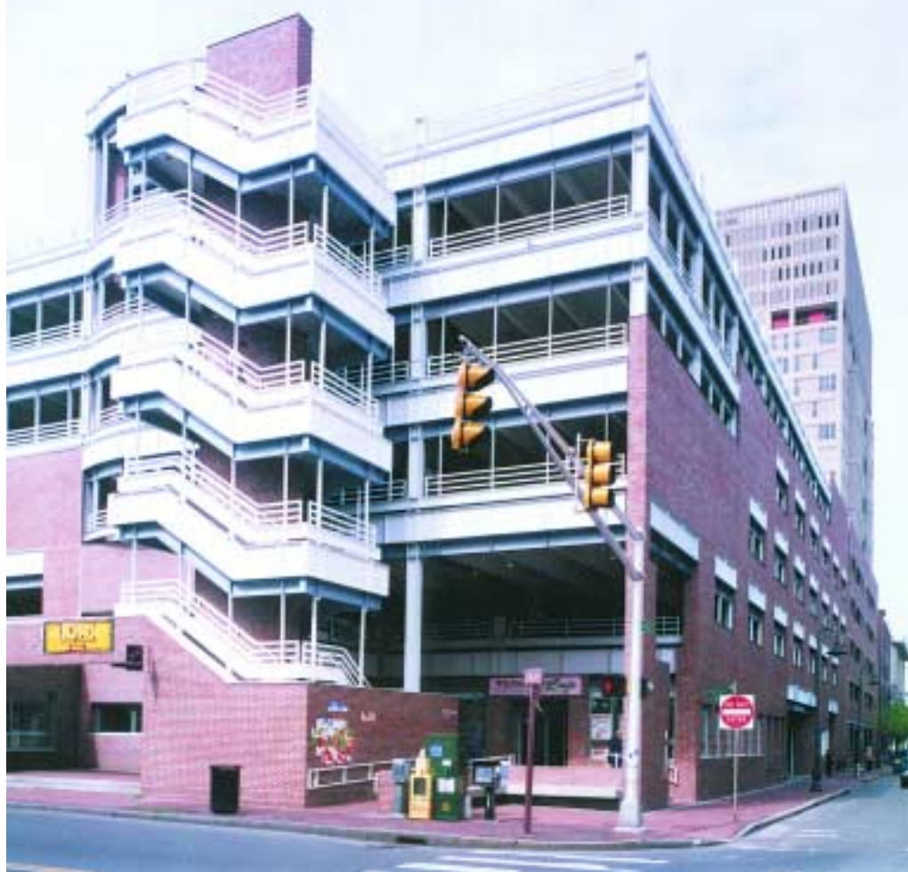
East Cambridge garage (Engineer: Hybrid Park- ing Solutions)
