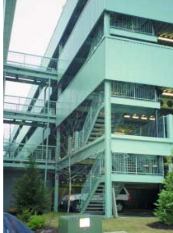
Corner view at stairs.
