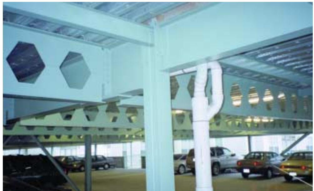
View of column and interior girders.
