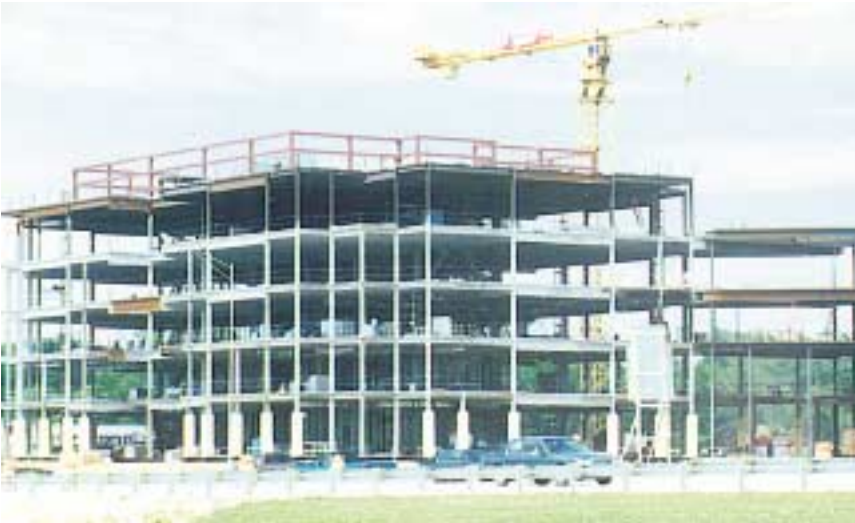
Structural steel erection in progress.
