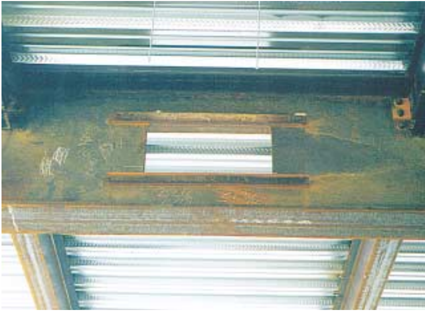
Beam web opening for duct.
