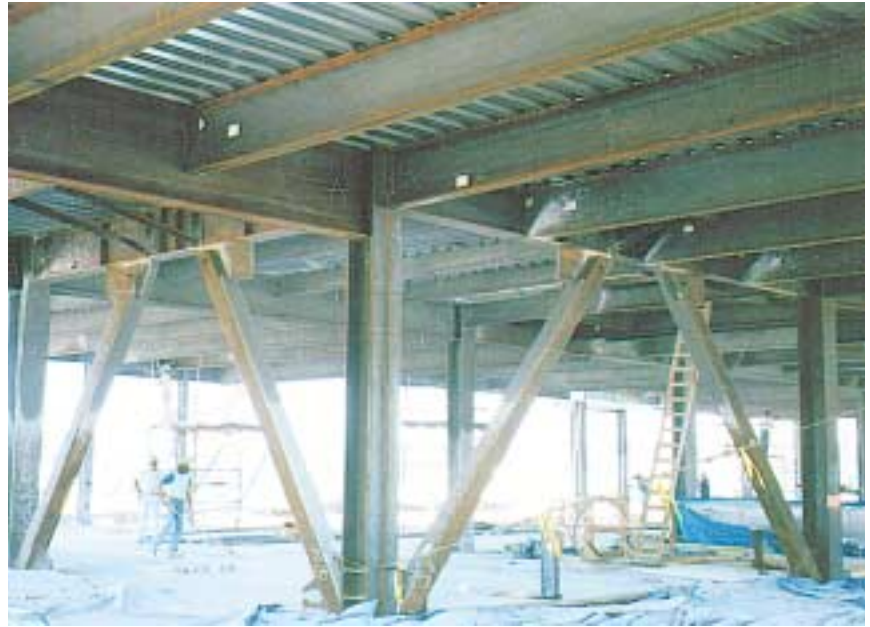
Eccentric braced frames.
