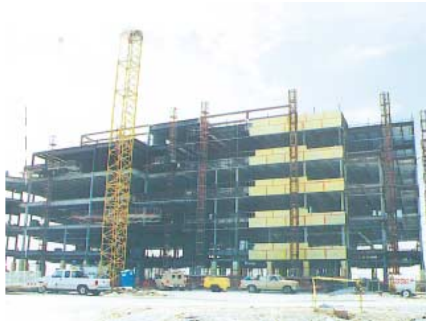
Brick spandrel frames.
