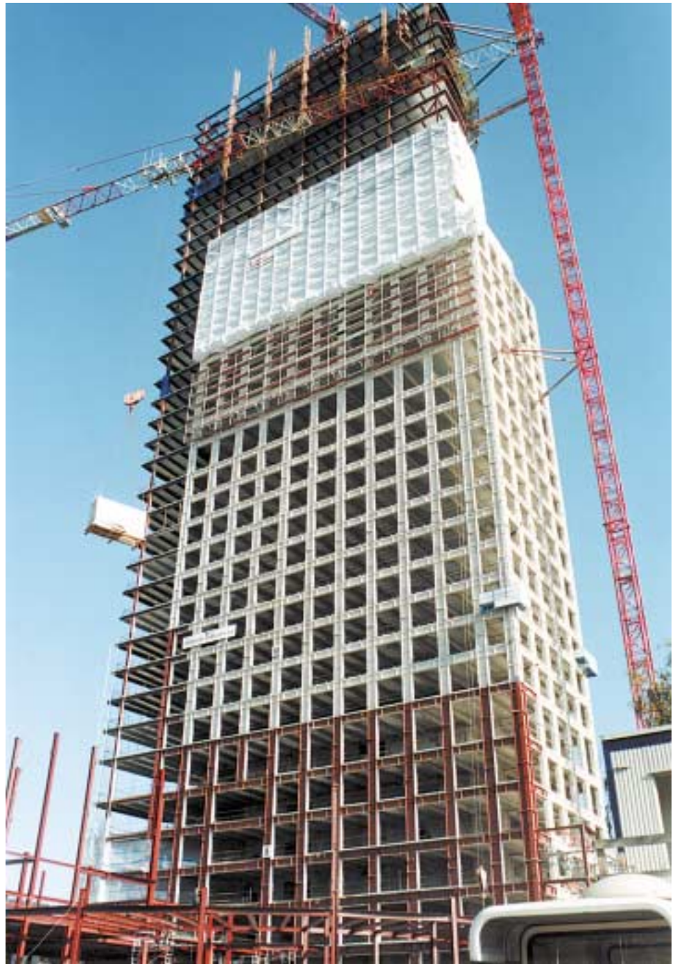
The Warsaw Daewoo Center nearing topping out.
