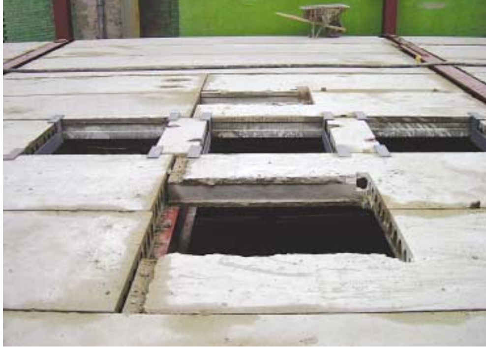
(top) Large mechanical openings and skylights are framed out in the concrete hollow core planks.
