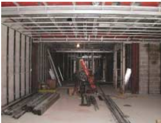
(top) Precast plank installed. Note the cut-out flange, lower right, that allows for the insertion of the planks, which are then slid into place. The flange cut-out, upper left in photo, is then welded back into place.
