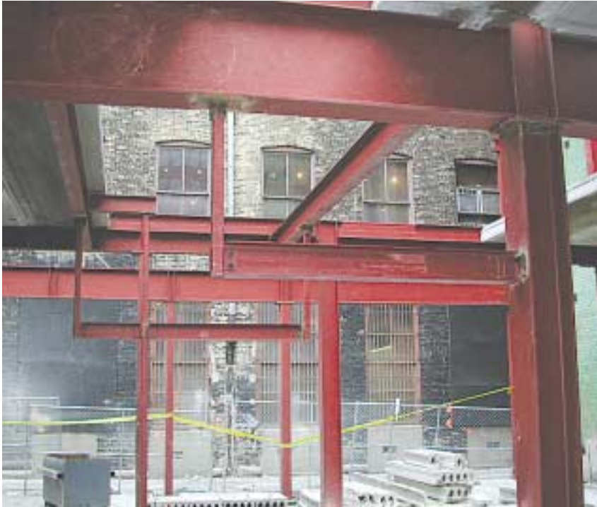
View at rear of first floor parking garage.
