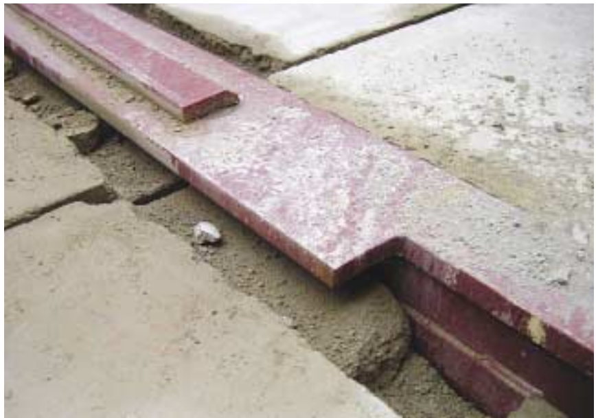
(top) Precast plank installed. Note the cut-out flange, lower right, that allows for the insertion of the planks, which are then slid into place. The flange cut-out, upper left in photo, is then welded back into place.
