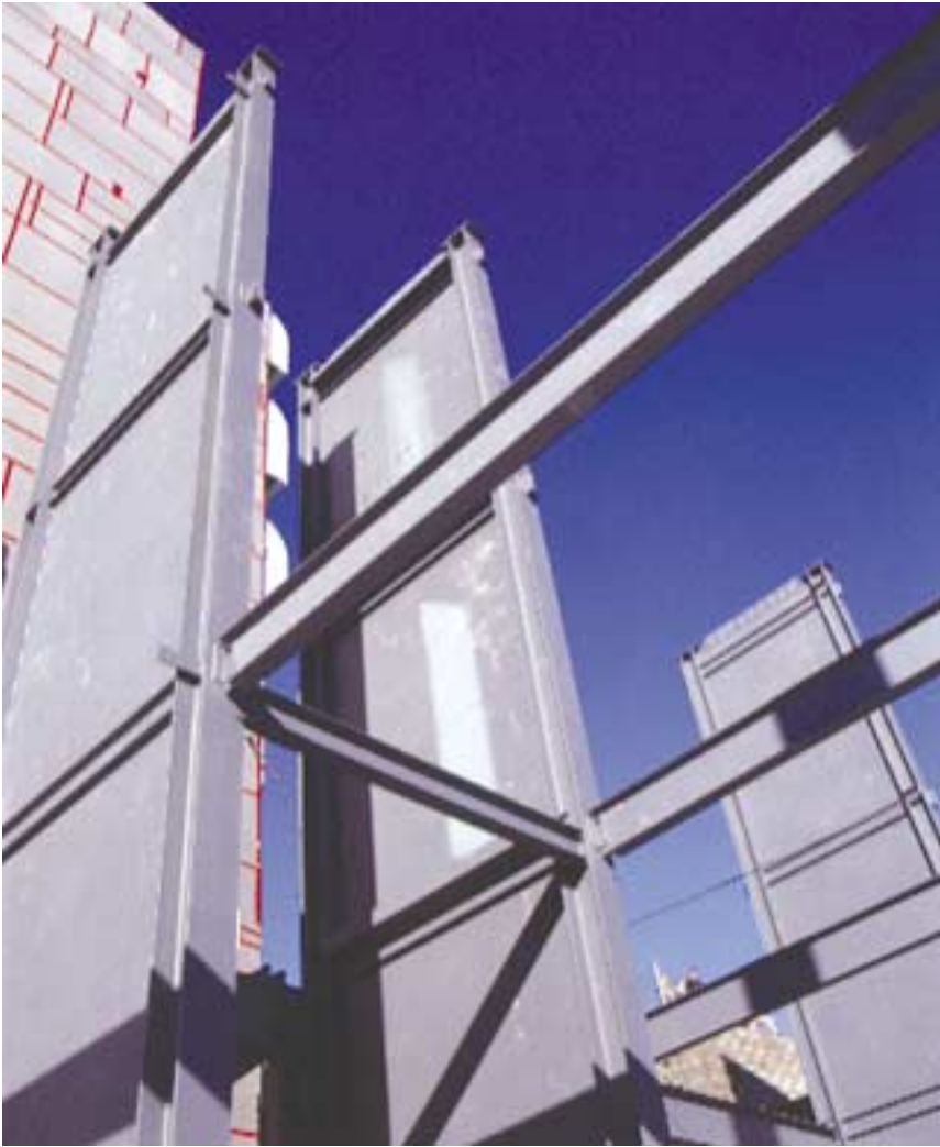
Figure 1. Steel plate shear walls (SPSW): Canam Manac Head Office Expansion.
