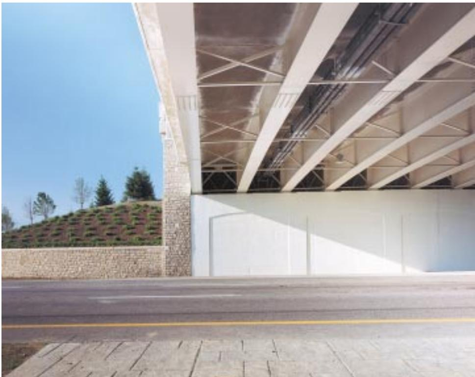
raise in profile grade on Avery-Muirfield Drive so as to avoid re-grading of interchange ramps that flank the bridge. It also needed to be easily constructed while safely maintaining all lanes of traffic both on and under the bridge throughout construction.
