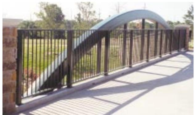
There is a 54" high steel handrail on each side of the deck. All of the steel structure and handrails are painted "Cedar Green." The concrete abutments and wing walls have a stone veneer.
