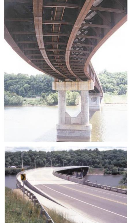
The first significant challenge was the transportation of the 4.3m (14') deep girders to the project site by water and train. The girders were fabricated by PDM Bridge, of Eau Claire, WI. It took an enormous amount of manpower, equipment and coordination to accomplish this task. Another difficult challenge was the fabrication and erection of these same large girders. This task was also difficult because of the tight radius of 155m (509') in the curved section of the bridge.
