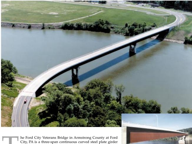
bridge with a total length of 323m (1060'), carrying S.R. 0128 over the Allegheny River and the Pittsburgh and Shawmut Railroad . The structure showcases Pennsylvania's longest curved girder to date and PennDOT's first use of grade 485W (70 ksi) high performance steel.
