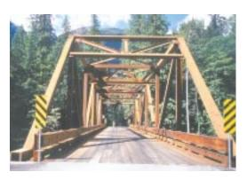
An engineering consultant was contracted to assist in preparing design visualization sketches to convey the concept to the park. The replacement bridge was to be a one-lane, six-panel Warren truss bridge made from unpainted weathering steel. Glue laminated timber deck panels and bridge rail were chosen to complement the texture and feel of the truss.
