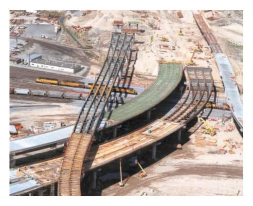
bracing resulting in more economical fabrication and material purchase. A welded full depth plate type diaphragm was used at the pier and abutments.
