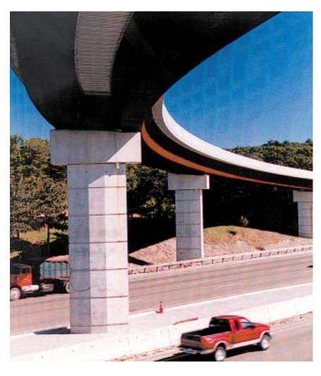
he I-93 Industriplex interchange project was the first fully directional T-interchange in Massachusetts. Based on type studies, VHB chose curved twin steel trapezoidal boxes to meet tight curvature and minimize structure depths. VHB partnered with the contractor for development of erection procedures. Erection over the Interstate (vpd = 120,000) incorporated southbound closure and northbound crossover. Erection of the girders was completed in less than 36 hours over the weekend.
