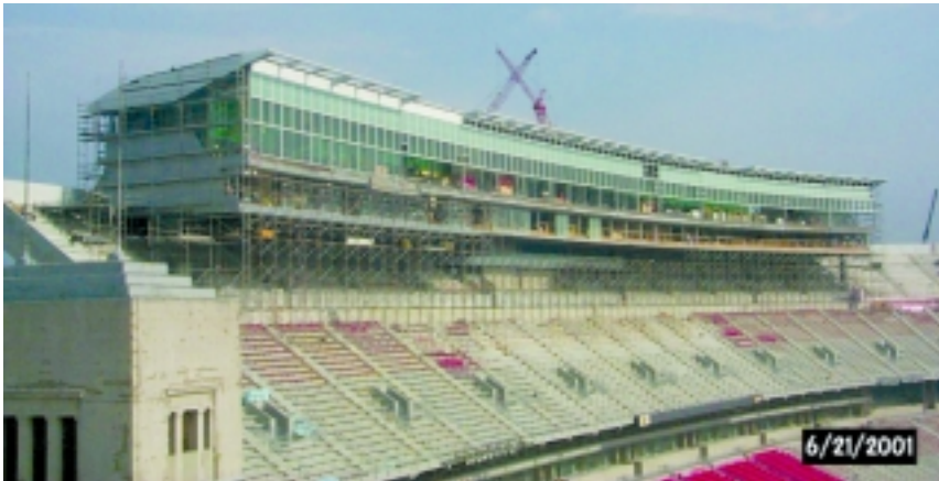
Partially-enclosed press box as viewed from the east.
