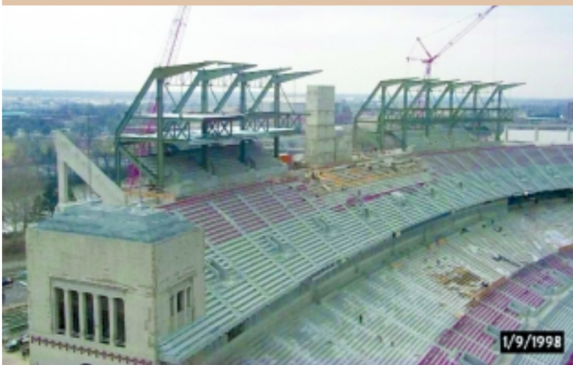
top: View showing ten of the thirteen frames erected. bottom: Four southerly frames. Note floor-to-floor truss at suite level.
