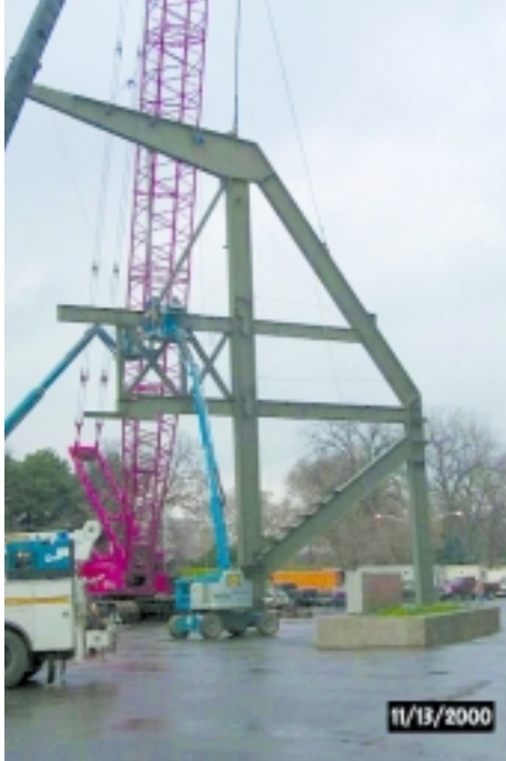
Pre-assembled bent frame being lifted into position.
