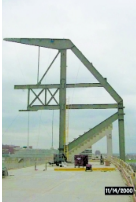
First erected frame on south end.
