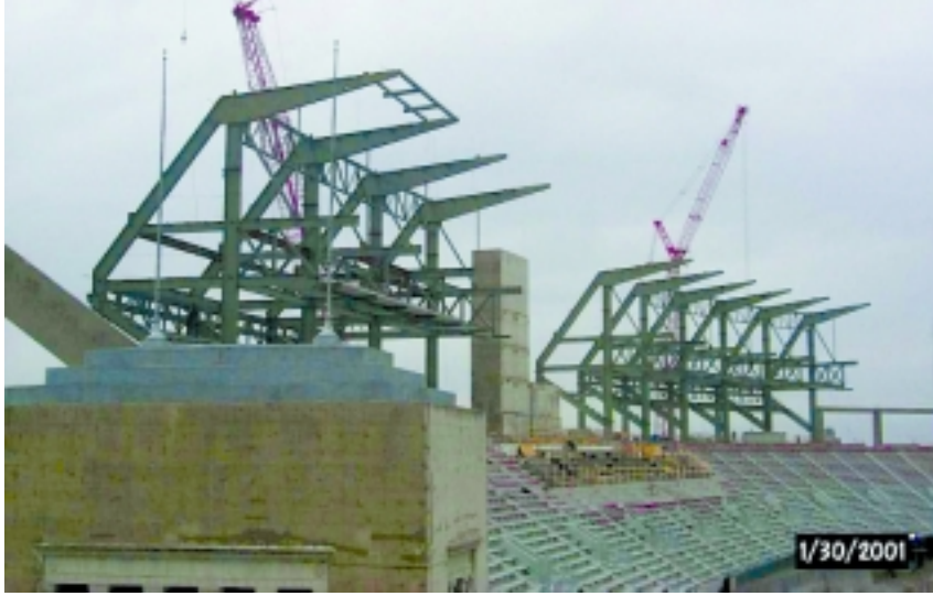
Existing press box demolition delays erection of center frames.
