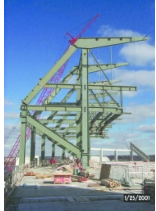
Typical frame as seen from the upper concourse.
