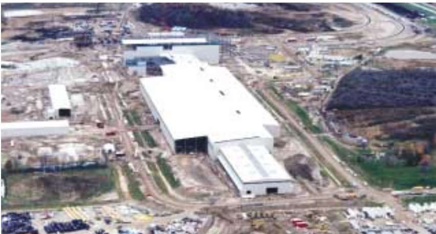
Aerial view of the new Steel Dynamics Inc. steel mill in Columbia City, IN.
