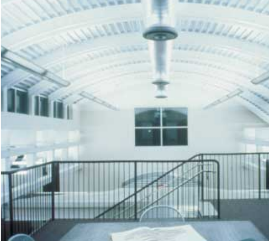
The upper conference room is supported on either side by the bottom chords of Vierendeel trusses made of HSS.
