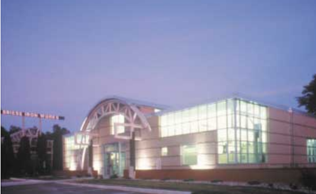
An early evening view of Briese Iron Works shows the extensive use of exposed structural steel as a design element.
