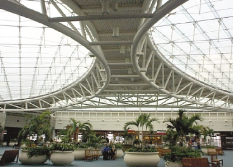
Architecturally exposed steel trusses and a tension cable truss skylight allows travelers to enjoy Florida's sunshine.
