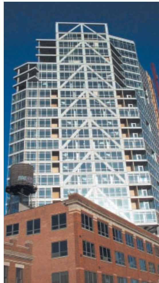
West elevation of 510 W. Erie. The steel and glass curtain wall stands out against the surrounding masonry buildings.
