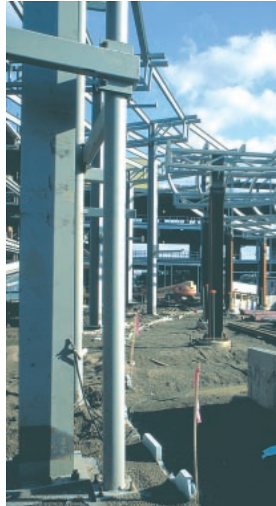
Steel frame for exterior canopy.
