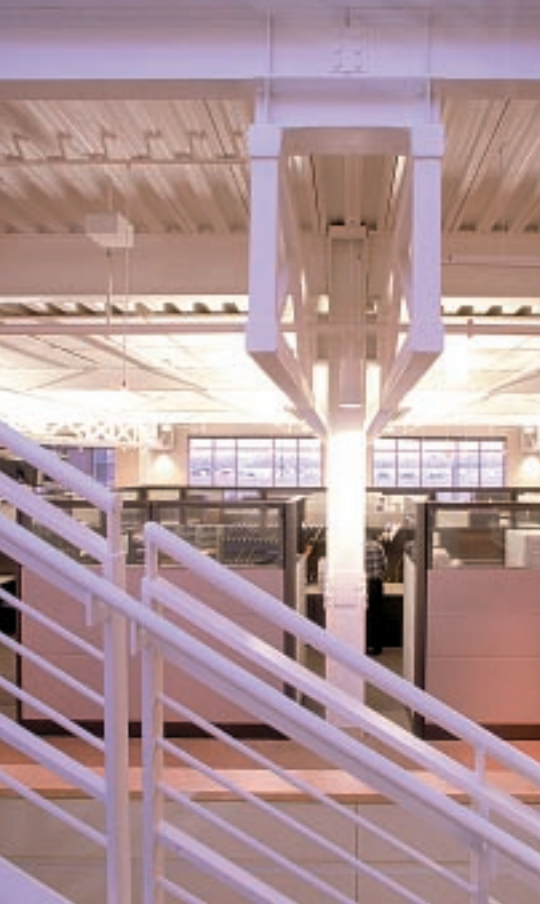
Custom-fabricated truss girders are located on each side of the column line.
