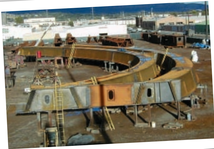
Structural steel was pre-assembled at the fabricator's yard to ensure a proper fit before it was trucked to Mississippi.
