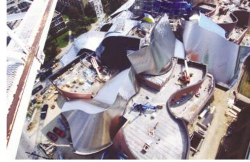
but the structural steel support structure for these surfaces required the design of two unique and never before used structural systems. The design and construction team referred to these systems as "ladder trusses" and the "stick and pipe" system.
