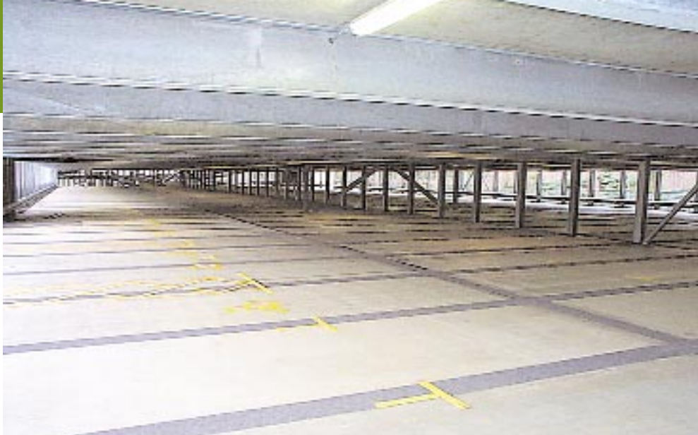
The Montex framing system provides a clear headroom of 2.2 m (7.2') and a floor construction depth of just 570 mm (22.5").
