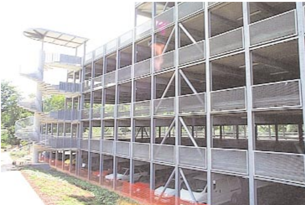
Steel framing creates a light, airy structure.
