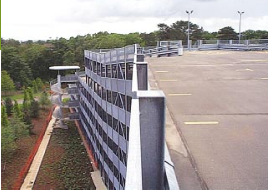
Galvanized steel framing provides durability.
