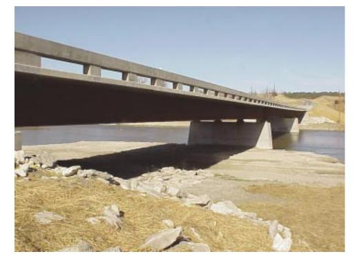
Integrating highperformance 70 ksi steel (HPS) with traditional 50 ksi steel yielded a design that cost 10% less than the lowest concrete bid.
