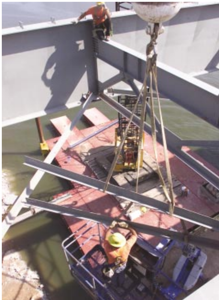
Workers install lateral bracing for the girders.
