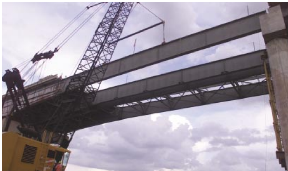
The last bridge girder is lifted into place.
