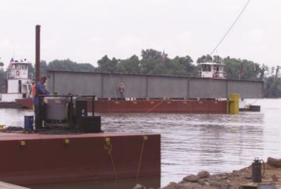
The last girder is transported to the job site.
