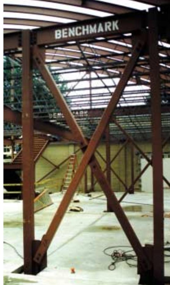
Conventional X-bracing using HSS and angle shapes was used to provide lateral stability for the addition.
