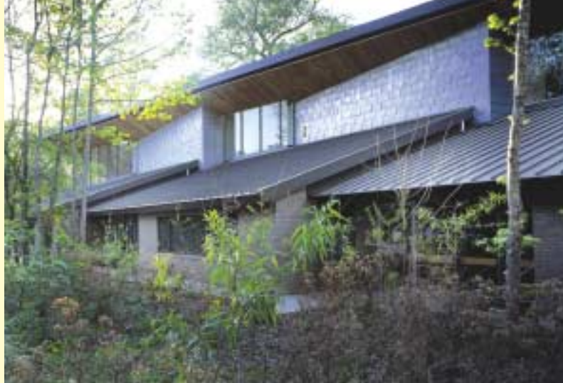
Above: The rear of the building is broken into smaller scale units reflecting the pattern of its use. All of the exterior cladding materials—brick, metal siding and metal roof—were colored to reflect colors found on the site.
