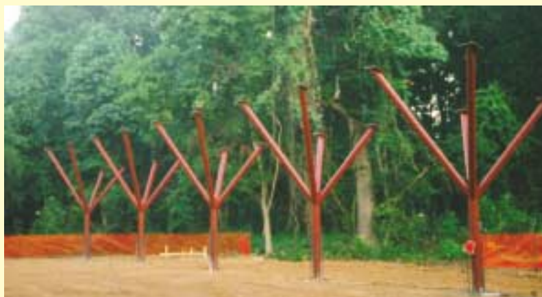
Below: The steel “trees” are set into 16 ft-deep drilled shafts that were then filled with concrete.
