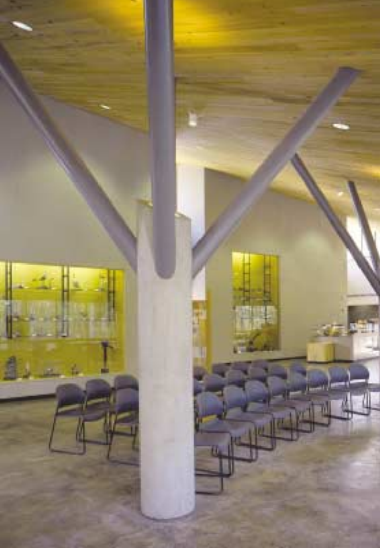
Above and opposite: The steel “trees” provide a dramatic sense of uplift within the exhibition gallery. The steel trees provide both drama and crucial moment resistance while reflecting the forms of the Louisiana oil industry.
