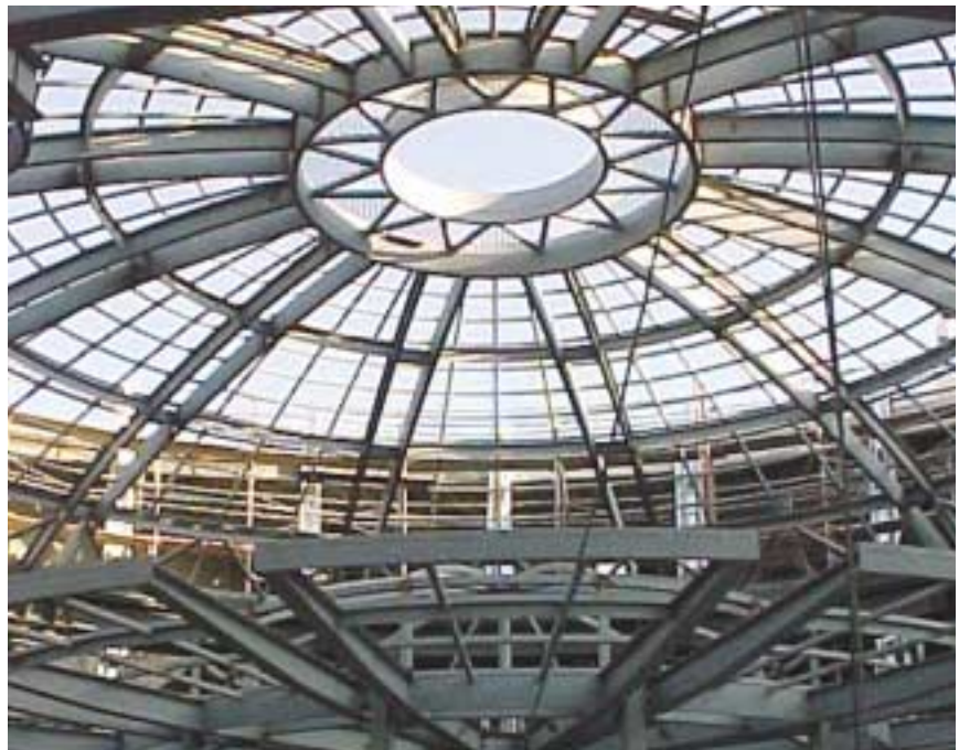
The ribs of the entry dome consist of double-channel sections that reduce member depths and provide visual interest.
