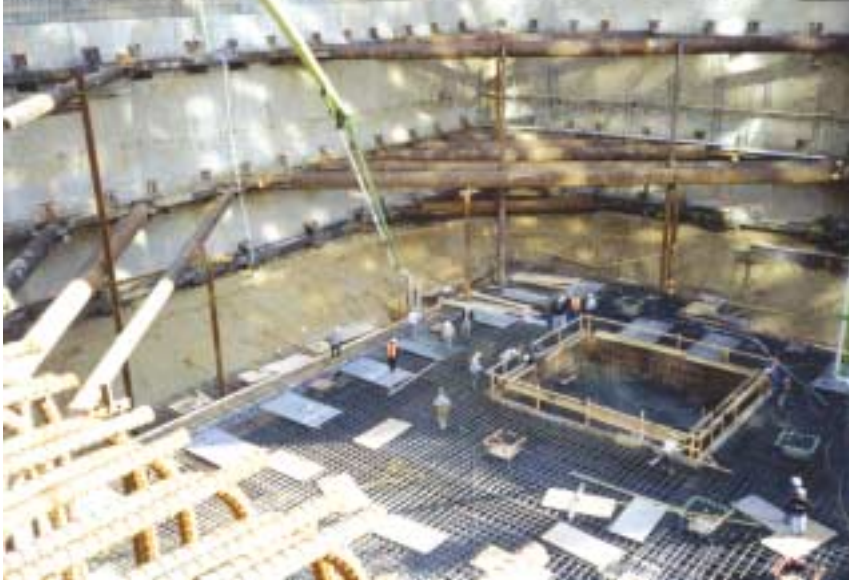
24" diameter extra-strong steel pipe cross-lot braces with W36×182 spreaders were used for the lateral support of the slurry walls during excavation.
