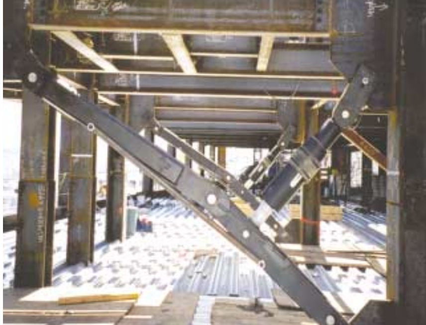
Construction photo of the bent-knee toggle damper assembly. Note the deviation angle of the main diagonal struts.
