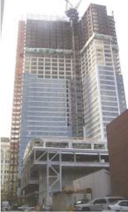
Photograph of the rear of the building during construction. The irregular "boot" shape of the structure is evident from this angle. Also shown are the cantilevered ballroom and basketball levels as well as the three story voided area for the future museum.
