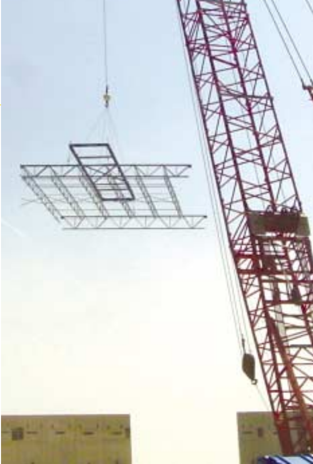
Above: By pre-assembling joists in bays, the structural steel erection process progressed more efficiently and reduced chances of worker injuries during construction. The erected steel shell for the facility was in place in only 4½ months.
