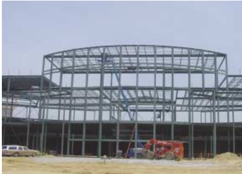
Above: By pre-assembling joists in bays, the structural steel erection process progressed more efficiently and reduced chances of worker injuries during construction. The erected steel shell for the facility was in place in only 4½ months.
