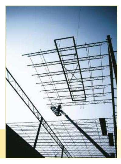
Opposite page: Bratton Steel assembled panels for the Nebraska Furniture Mart in Kansas City, KS for a week before they were erected. In this photo, erectors raise a panel from the stack in preparation for hanging.
