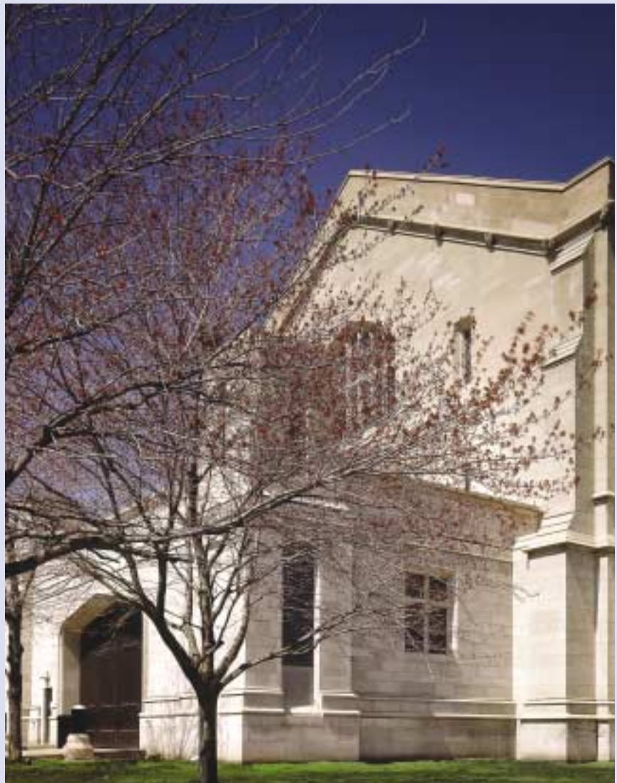
Below: Although clad with limestone veneer rather than solid limestone masonry, the loading-dock addition blends seamlessly with the existing building because of careful detailing.
