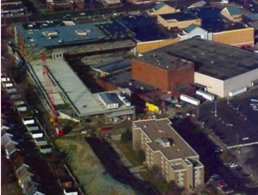
A two-level department store was relocated to make way for the steel-framed parking structure.
