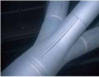
HSS cast steel node.
