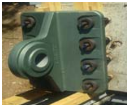
Above: Cast steel cable anchor for the Max Eyth See bridge near Stuttgart, Germany. Below: Pedestrian bridge in Bayreuth, Germany with cast steel cable clamps.
