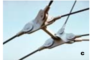
Roof for the 1972 Olympics in Munich, cast steel nodes for cable coupling. a) Roof; b) Foam model; c) Final installation of cable coupling.
