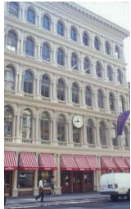
Cast iron façade, Haughwout House, New York.
