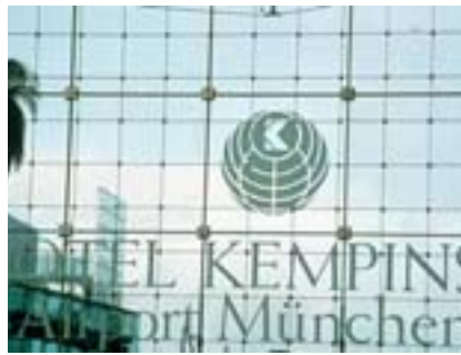
Cable net façade for the Hotel Kempinski in Munich with stainless cast steel corner patch plates and cable clamps.
