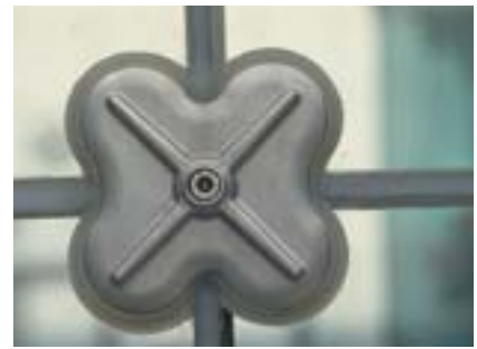
Cable net façade for the Hotel Kempinski in Munich with stainless cast steel corner patch plates and cable clamps.
