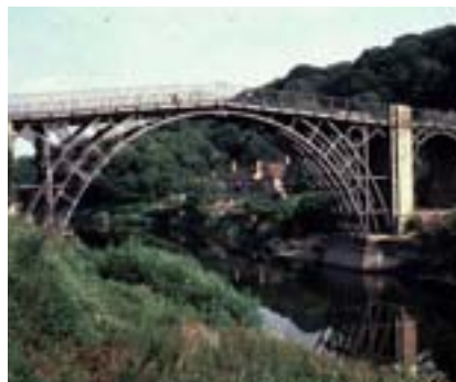
The first cast iron bridge, Coalbrookdale, England (1777–1779).
