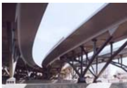
Railway bridge across the Humboldthafen.
