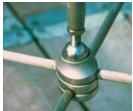
Left and above. Courtyard roof of Deutsche Bank, Berlin with cast stainless steel cable clamps
