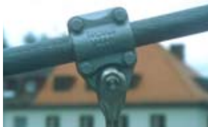
Above: Cast steel cable anchor for the Max Eyth See bridge near Stuttgart, Germany. Below: Pedestrian bridge in Bayreuth, Germany with cast steel cable clamps.
