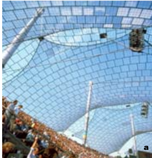
Roof for the 1972 Olympics in Munich, cast steel nodes for cable coupling. a) Roof; b) Foam model; c) Final installation of cable coupling.
