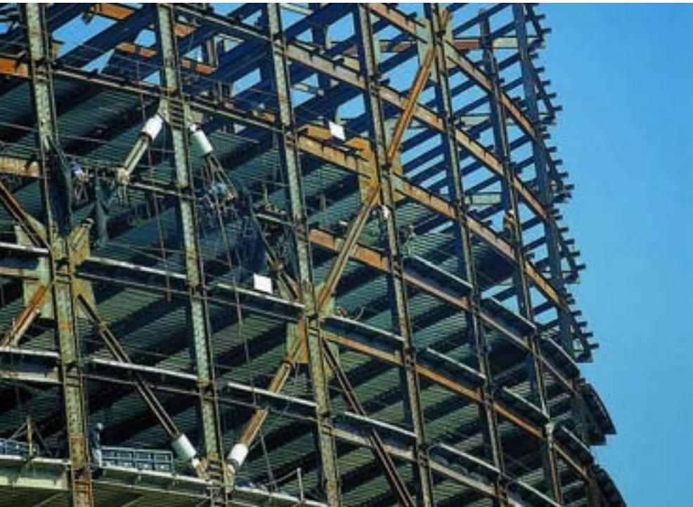
Lateral bracing forms a super-X configuration on the east and west faces, where the X covers the entire width of the tower. On the north and south faces, two sets of super-Xs were introduced.
