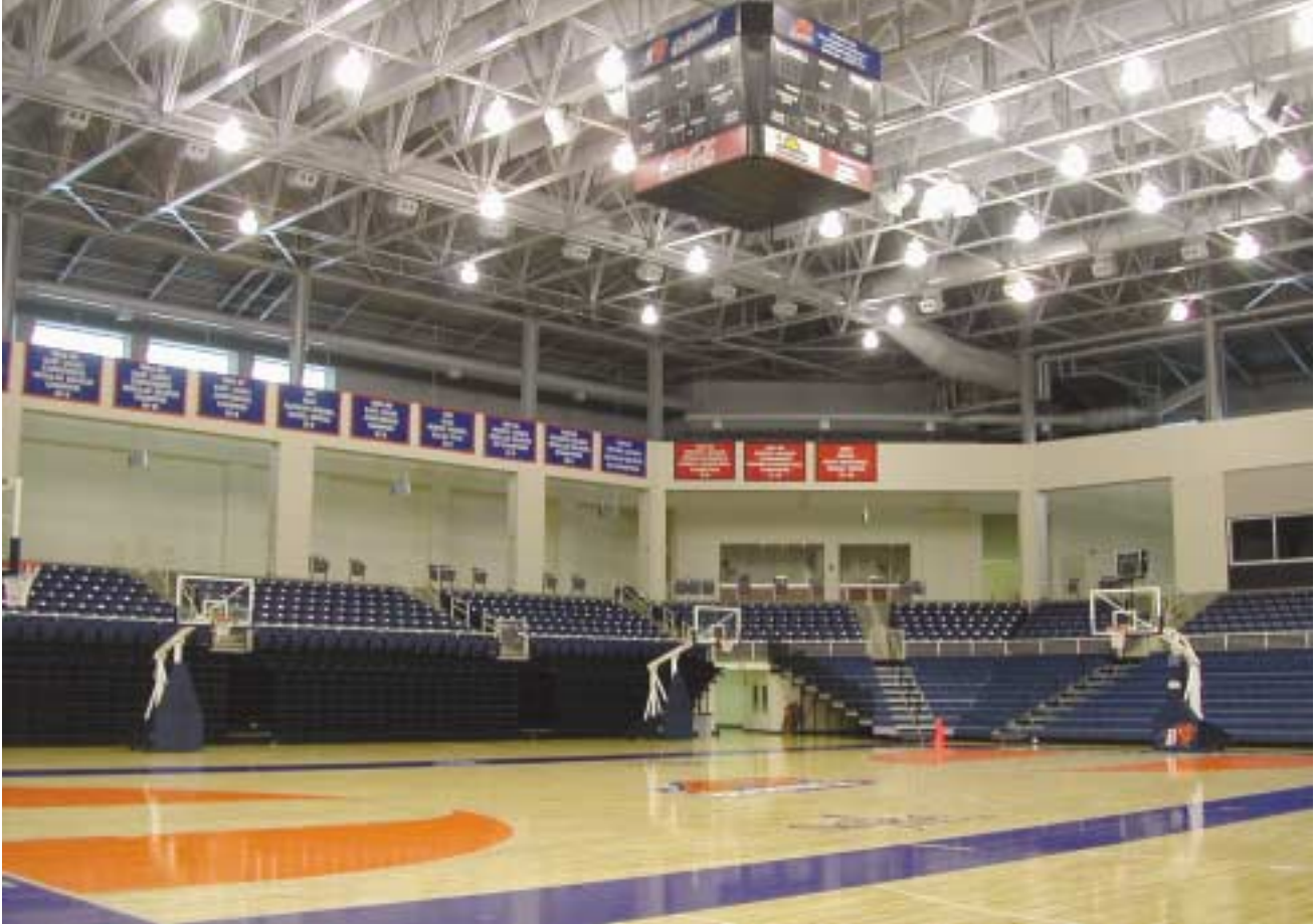
Exposed long-span-joist roof and center-hung score board in gymnasium.
