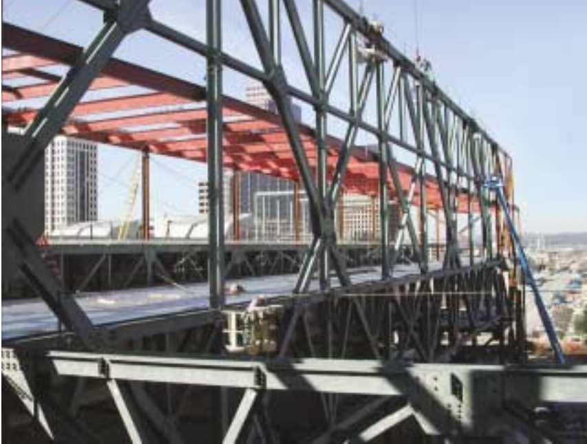
The 65'-deep super-truss spans 270'.
