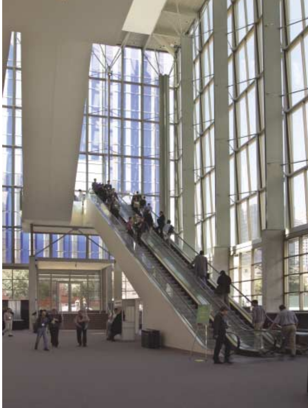
Within the glass pavilion, the escalators run to an intermediate landing adjoining a cantilevered balcony.
