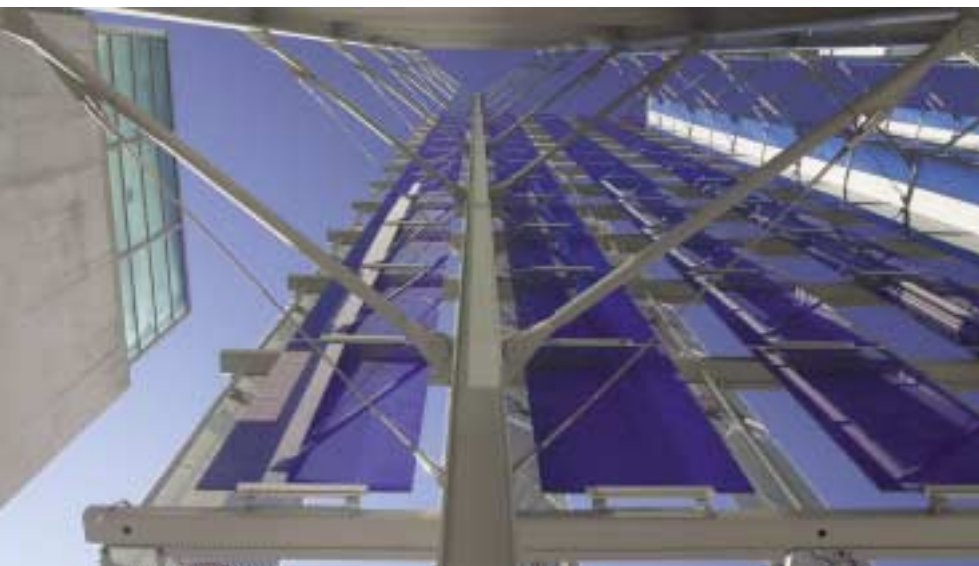
The exterior "art wall" uses panes of cobalt-blue glass supported by structural steel struts to filter sunlight into the atrium.
