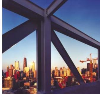
rie on the Park is a striking statement in steel. This sleek 25-story residential tower emphasizes the material with exposed chevron-shaped steel bracing punctuating the façade. The result is a distinctive design that stands out in the Chicago cityscape, where concrete is the typical choice for apartment buildings. Floor-to-ceiling glass runs between steel spandrels and the dramatic chevrons, achieving an open airy look and offering building residents views of nearby Lake Michigan.
