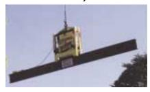
The CONNECTOR™, a self-contained, hydraulic-motor-driven lifting clamp, was developed to address positive load control and OSHA fall-protection requirements. Certified for a safe working load of 11,000 lbs, the device safely picks and transports beams, bar joist, and other structural materials to the delivery point, and then enables unhooking without workers having to go onto the suspended load.
