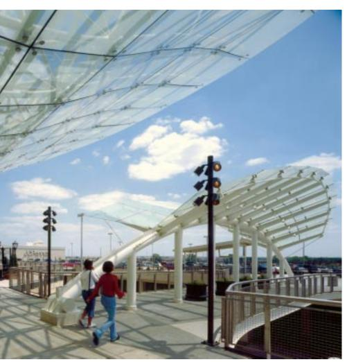
then raised up along its edges. Constructed using a series of king-post trusses assembled from wide-flange steel top chords, HSS compression struts, tension rods, and steel rod bracing, the undulating roof bears lightly on a diagonal HSS truss framing the clerestory glass.
