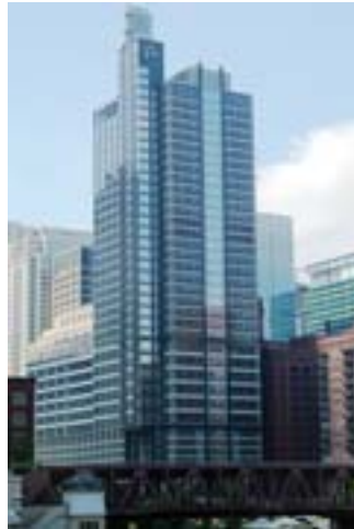
The Boeing Building, 100 N. Riverside, Chicago. The low-rise portion (lower left in photo) is cantilevered over active railroad tracks.
