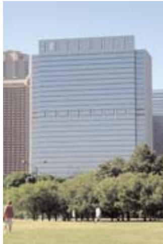
The Blue Cross/Blue Shield Building, 300 E. Randolph St., Chicago, is designed for vertical expansion without disrupting current tenants.
