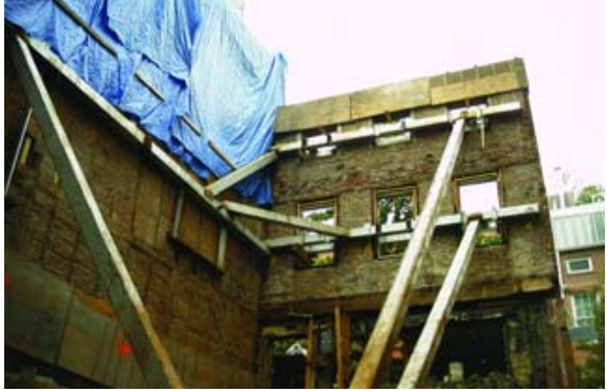
Because of the constraints of the site and the fragility of the historic construction, structural steel bracing was installed from a temporary concrete footing in the center of the building before demolition of the rest of the structure.
