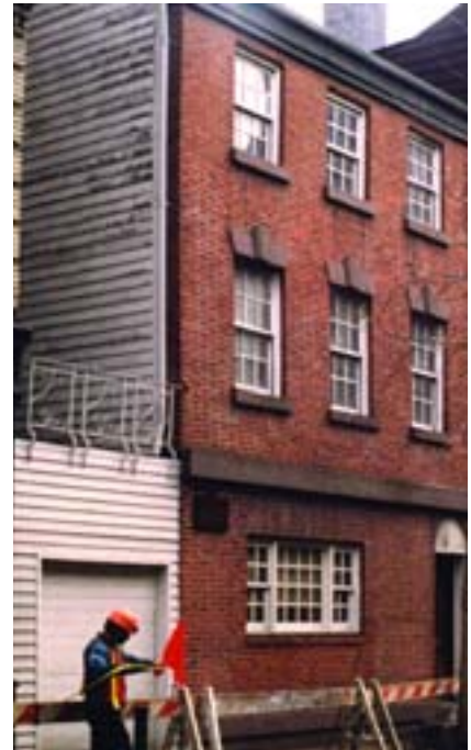
Built in 1806, the town house had been altered many times and was in poor condition prior to its reconstruction.
