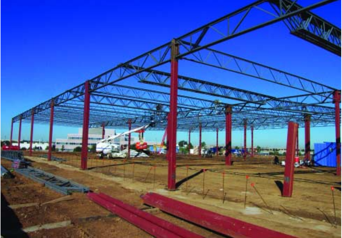
The roof structure for both buildings is composed of 26"-deep bar joists at 6' centers on 28"-deep joist girders. The one-story Building Two uses 8" square HSS columns.
